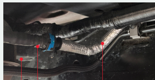
FIGURE 8A FUEL HOSE INSTALLATION - TANK END SIDE
